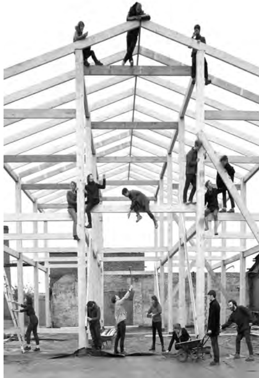
Figure 22 Assemble collective's Yardhouse studios for London creatives under construction
