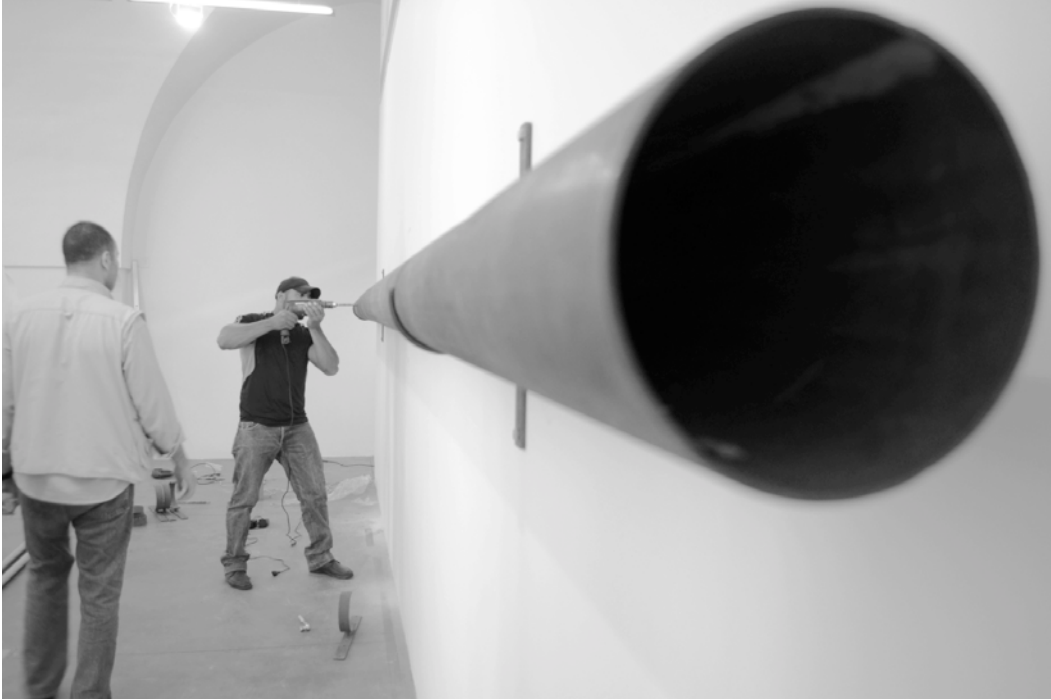
Exposed Pipe , Byblos Bank Art Gallery, Beirut Lebanon, 2013.
