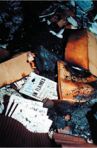
6200 Blackstone smoldering after a suspicious fire gutted the building April 25th, 2001 and close-up of burnt copies of The Baffler from inside the building.
